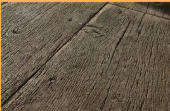
Gilpin Falls Bridge Plank
